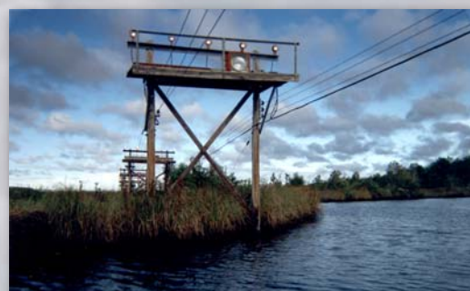
Hancock Creek next to Runway 32L approach lights
